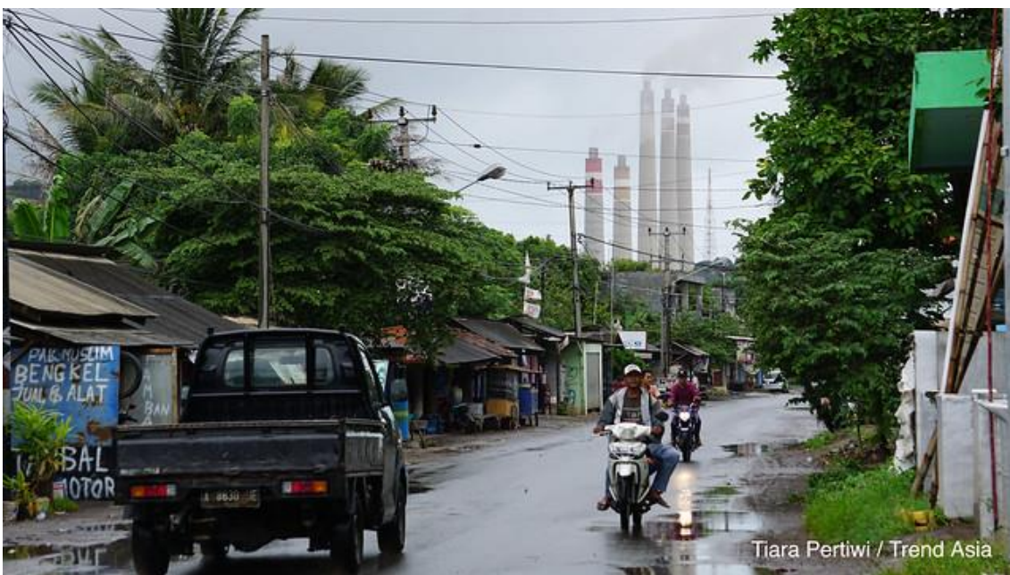
Existing units of Banten coal power plants looming over the residents of Banten Suralaya
